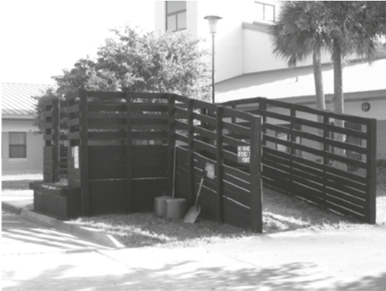
Figure 1.8 A loading ramp should have tall sides and good footing. Source: Courtesy of Dr. Dana Zimmel.
